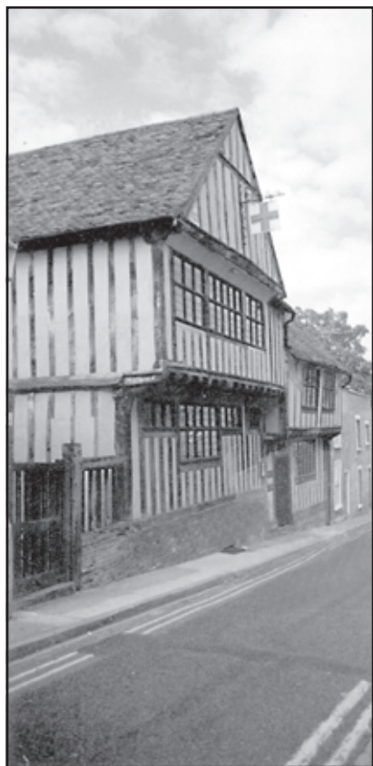
Houses with the second floor overhanging the first
